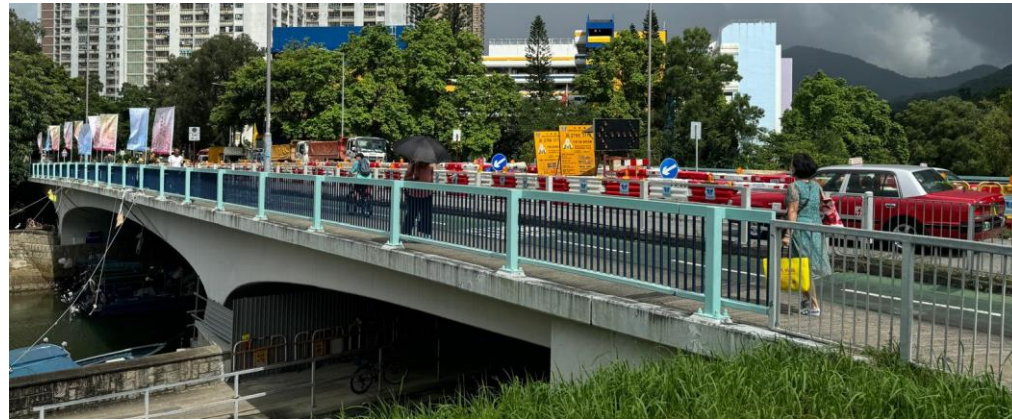
Pedestrian and vehicle bridge
